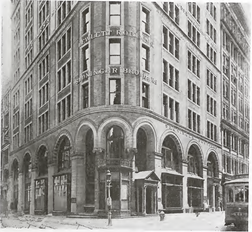
FIG. 3. BROADWAY, S. E. COR. OF 20TH STREET.
